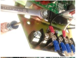
Secure new TRIAC with #6-32 x 1/2" Screw and Nut with Lockwasher using 5/16" Wrench and #2 Phillips Screwdriver
